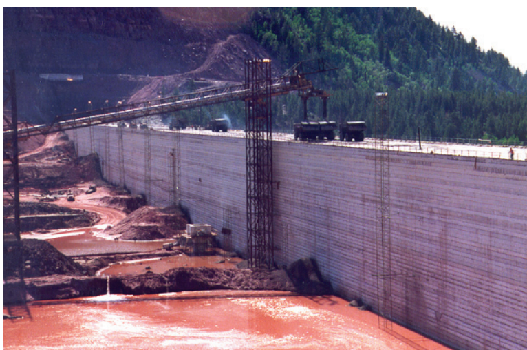
Fig. 4. Upstream face of Upper Stillwater Dam during construction
