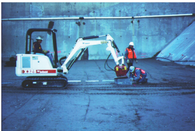
Fig. 5. Installation of crack inducer at contraction joints
