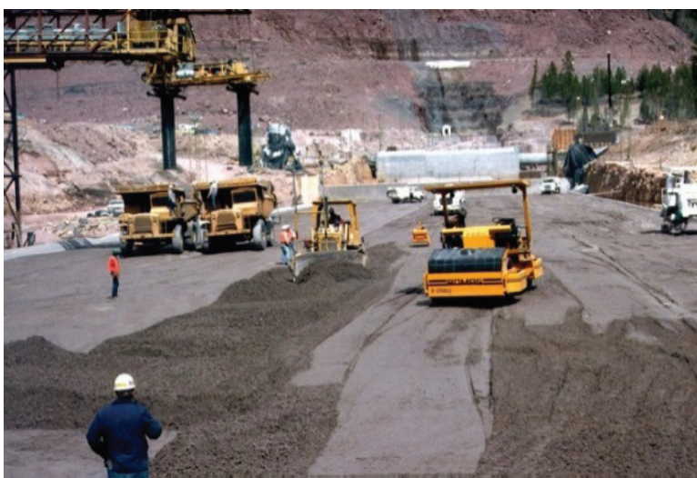
Fig. 3. RCC placement - spreading and compaction process
